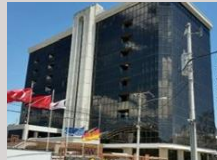
Torre La Sabana, 12,394 M2, San Jose, Costa Rica
